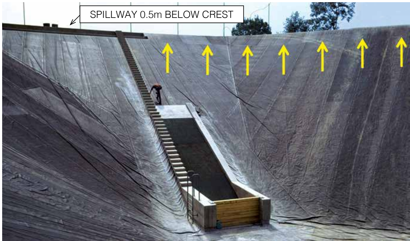
FIGURE 3 Southwest end of the reservoir showing: water intake structure, spillway, and butyl rubber geomembrane. The butyl rubber geomembrane is unreinforced, except at the top of the slope where a strip of reinforced butyl rubber geomembrane is used around the entire perimeter (except at the spillway) above the level marked by the yellow arrows and in the anchor trench.
