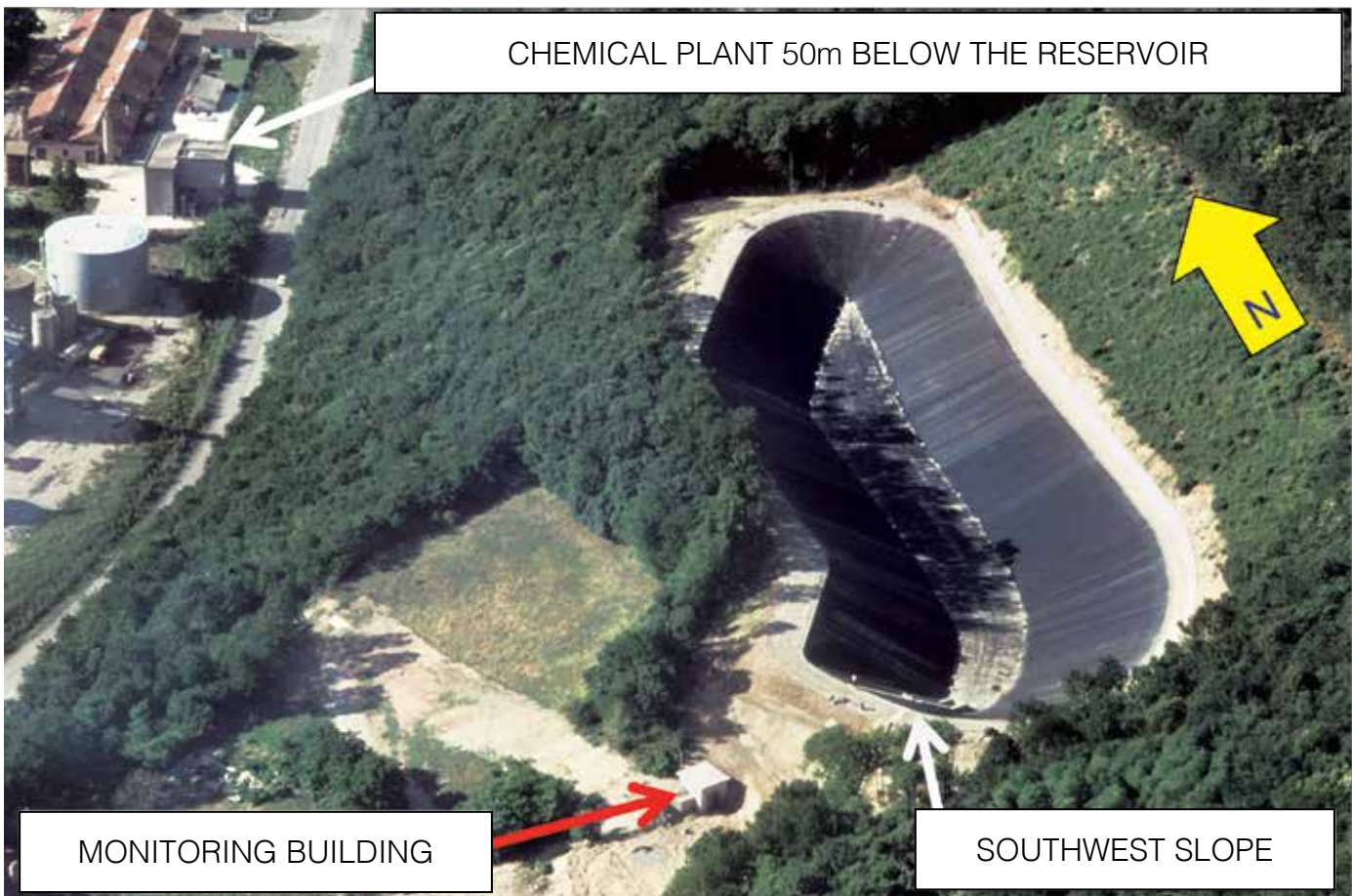
FIGURE 2 Aerial view at the end of geomembrane installation. The shape of the reservoir minimizes the impact of excavation on the stability of the east slope and the weight of the dike on the west slope. The reservoir proportions are distorted because the photo was taken at an angle (as evidenced by the fact that the intake structure on the 1V:2H southwest slope is hardly visible).
